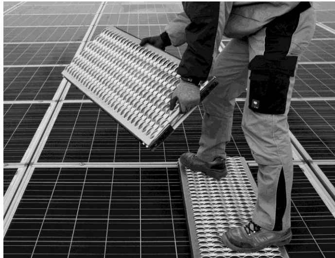
Figure 7: Installation of SMB SOLAR MULTIBOARD
