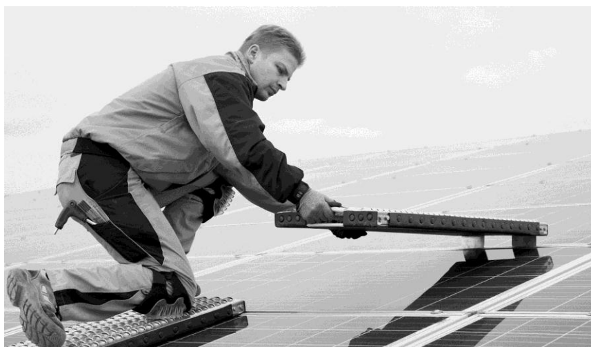
Figure 8: Inserting the SMB SOLAR MULTIBOARD
